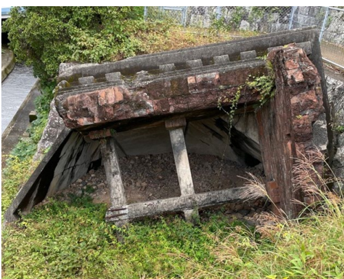
Urakami Cathedral Belfry blasted off the Cathedral and coming to rest down the hill adjacent to the Cathedral.
